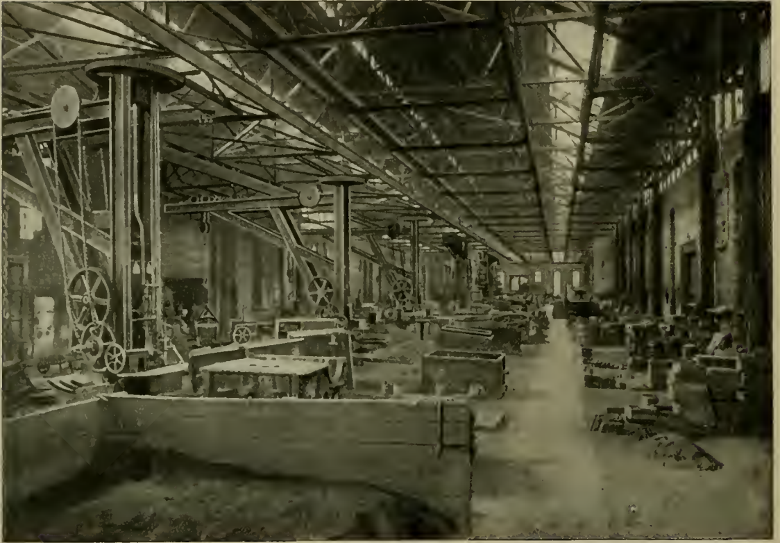
IN THE FOUNDRY—BALDWIN'S.
